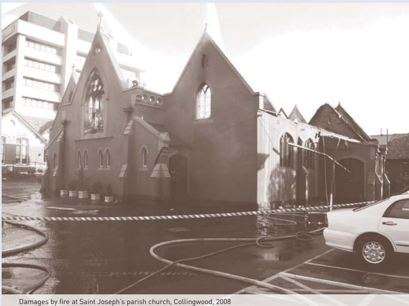
Damages by fire at Saint Joseph's parish church, Collingwood, 2008
