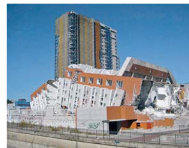
Figure 8. Fully collapsed building located in Concepción (Source: AIR)
