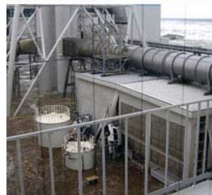
The following sequence of photos were taken from the 4th floor of the waste processing building at the power plant. They were shot over the course of a minute and reveal how quickly the tsunami inundated the area. Source: TEPCO
