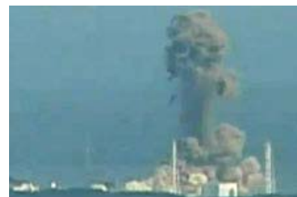
Figure 8. Highly energetic vertically propagating hydrogen or possibly steam explosion at the Fukushima Daichi unit 3 BWR on March 14, 2011 was followed by a fire and suspected reactor fuel damage. Heavy debris possibly composed of the concrete shield plug or crane components was vertically ejected and is seen falling back down in the photograph. No damage to the reactor pressure vessel can be inferred
