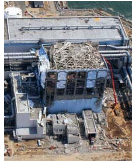
Figure 2. Aftermath of Fukushima Daiichi accident on March 18, 2011, one week after the accident. Rubble from hydrogen explosions in units 1, 3 and 4 is spread over the site. Damage from the earthquake and tsunami to the electrical systems is apparent along the water front. Steam still emanating from unit 2. Source: DigitalGlobe
